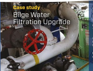
AW Ship Management needed improvements in bilge water oil content levels to enable overboard discharge. With the existing arrangement, the onboard oil-water separators struggled to meet the 15ppm legislation requirement.
